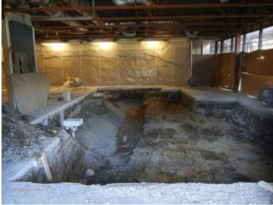
Excavation of the ground for the vibration isolation slab
