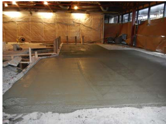
Completed vibration isolation slab (>100 tonnes of concrete).
